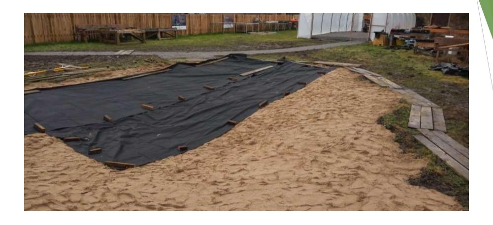
A layer of sand and protective material is hopefully enough to protect the liner against sharp stones left by the digging.
