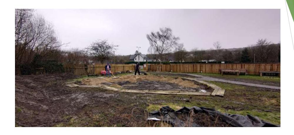
Sand layer going in to protect pond liner. Due to the site's industrial past, much of the substrate under the topsoil consisted of rubble and other porous materials. Therefore a pond liner was needed.
