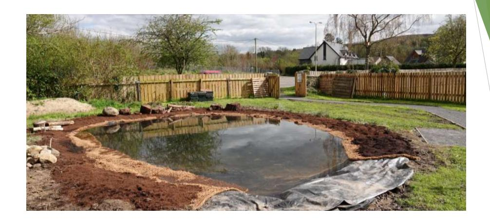
Pond liner trimmed and hessian laid around the pond, some peat-free compost added so the area can be seeded and in time blend naturally into the pond.
